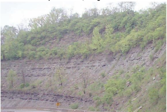
Shale and limestone in the Kope Formation in Kenton County (above) and Clark County (below). The shale content is greater than the limestone and this causes problems because it may become unstable and swell when wet. Top photo by Richard Smath, bottom by Dan Carey, Kentucky Geological Survey.
